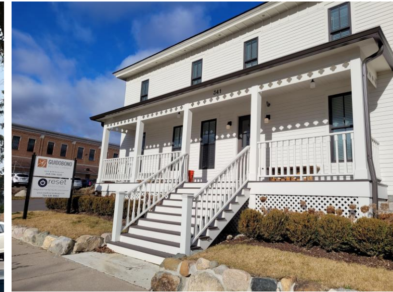
FORMER GOLD CURE BOARDING HOUSE
